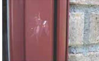
Large scrape on a casement window before being touched up. For repair on a larger area the foam brush technique usually provides the best results.
