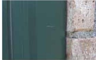
A small surface scratch shown on a picture window before being touched up using the applicator brush (included with the bottle of touch-up coating).
